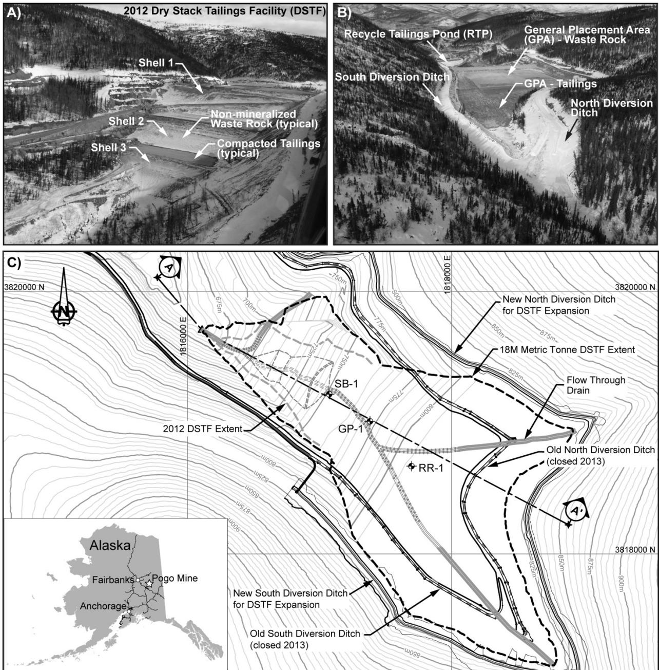
**Figure 1** Oblique air photo taken of the 2012 DSTF at Pogo Mine, Alaska: a) DSTF toe and composite shells, view facing up valley to east; b) general placement area, view facing down valley to west; c) plan view of DSTF
