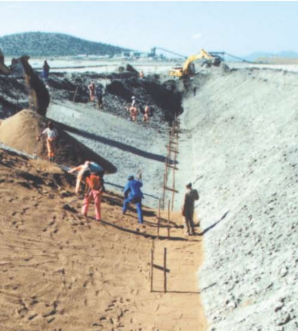
Continuous drainage installation as part of operation
