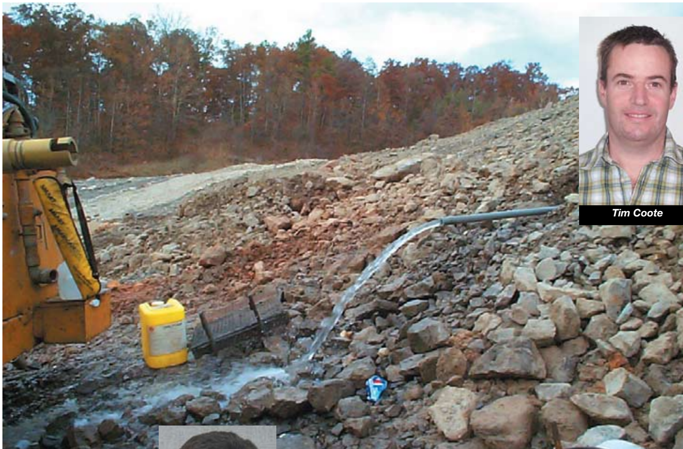
Brushy Creek Tailings Dam - Initial drain flow (DH-1) of 35 GPM
