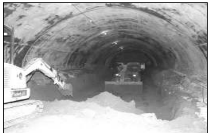
Fig. 3. Belgian tunneling method, Line H, 2000.
