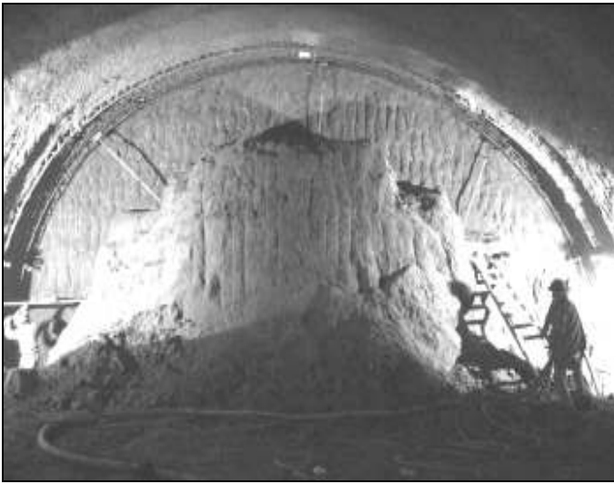
Fig. 4. Full face excavation, Line B, 2004.
