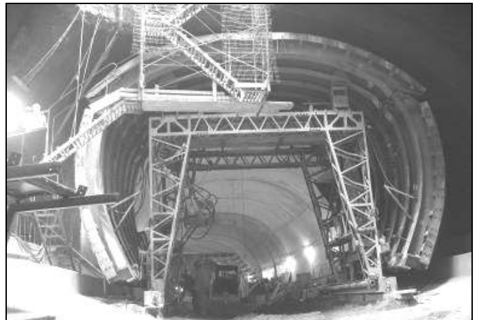
Fig. 7. Formwork used to cast the secondary lining, Line B.
