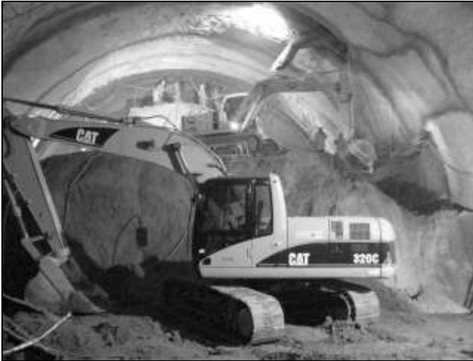
Fig. 9. Corrientes Station, Line H. Full face excavation.
