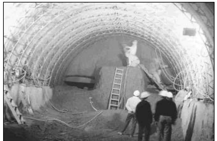
Fig. 2. First use of shotcrete, Line B.
