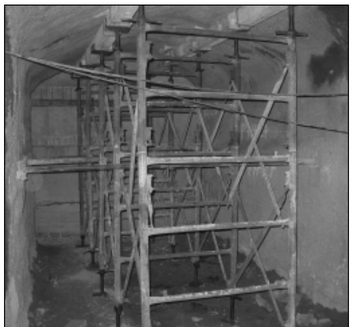
Fig. 13. Strut supported access tunnels, Echeverría Station, Line B.
