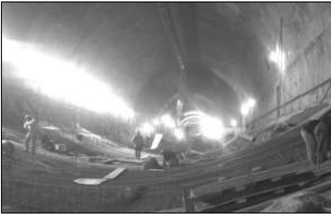
Fig. 8. Echeverría Station, Line B. German tunnelling method.
