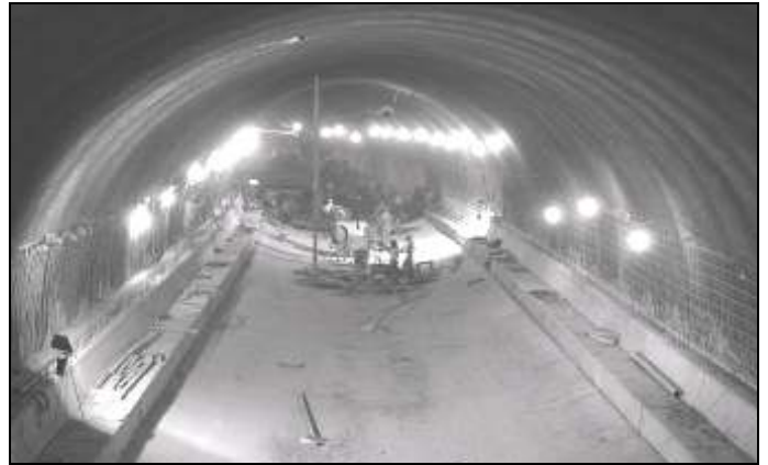
Fig. 6. Tunnel after placement of the invert, Line B.
