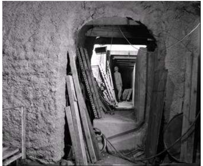
Fig. 12. Unsupported pilot tunnel for side walls, german method of tunnelling.
