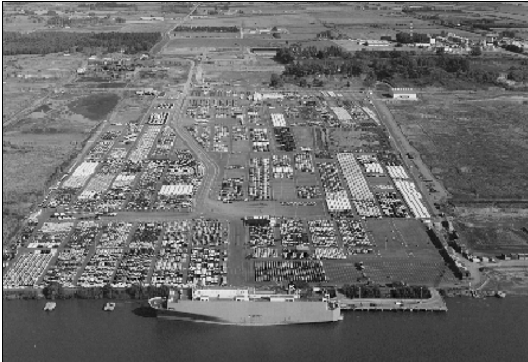
Figure 1. Aerial view of Autoterminal Zárate.
